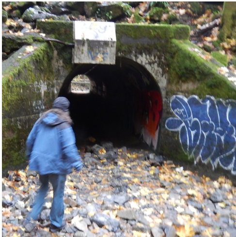
Goldstream Tunnel to the water fall
